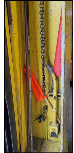
"I" beam with flags at South Entrance
